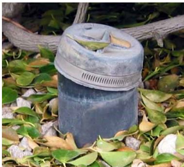
Examples of Pool Clean-Out Ports
