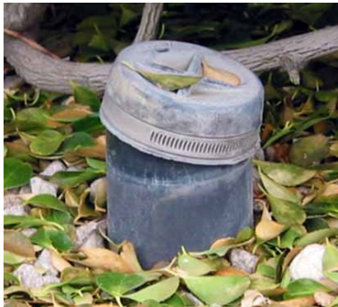
Examples of Pool Clean-Out Ports
