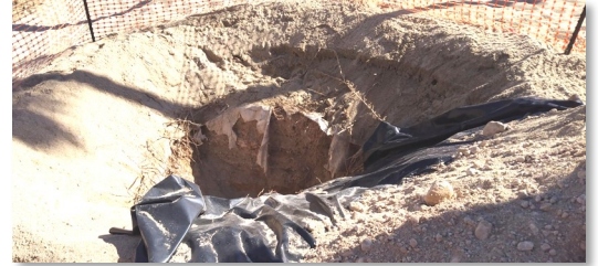
Digging & Prep work for the Palms
